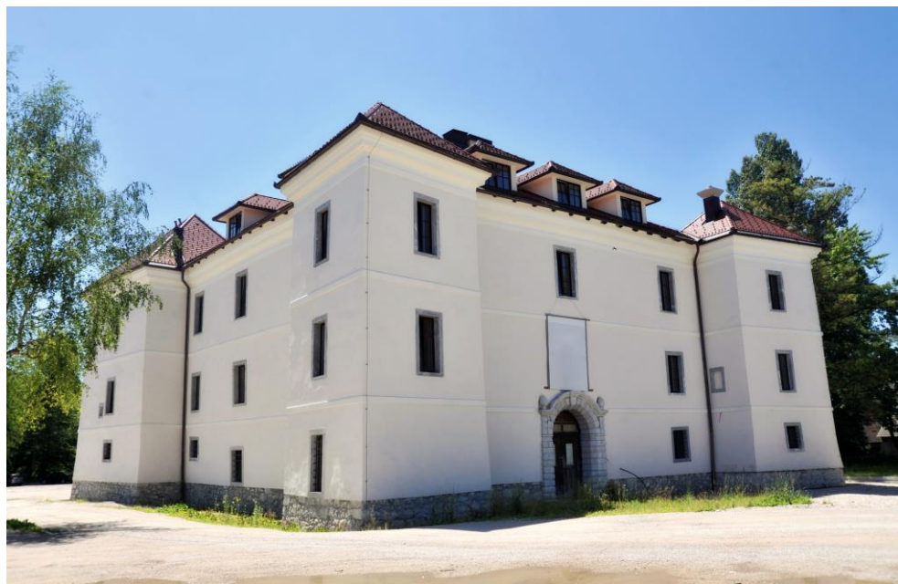
Fig. 11.25. Logatec Manor House.
